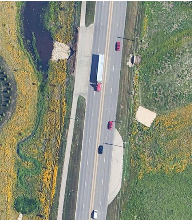
Figure 18. Truck Pullouts in Kane County, IL
